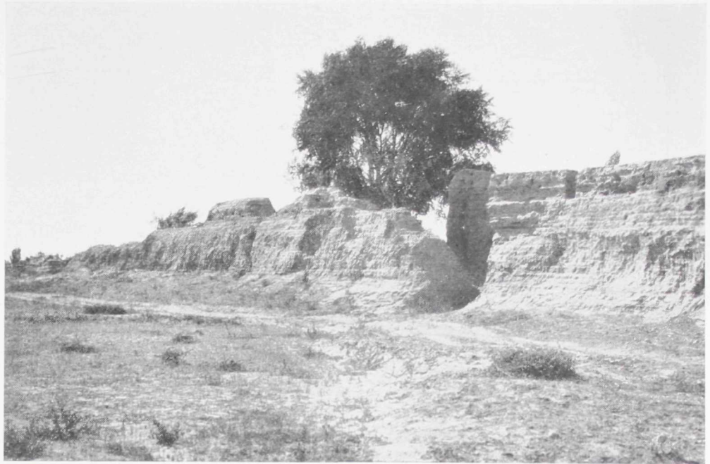
b. Part of the town wall of Meng-han-ch'eng
