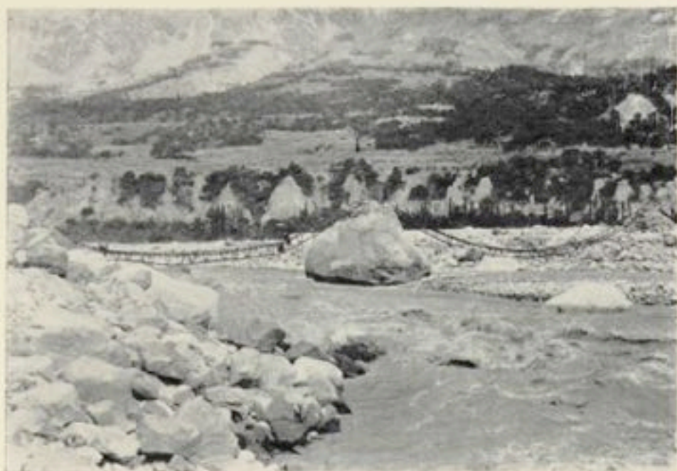
BRIDGE OVER NAGIR RIVER
