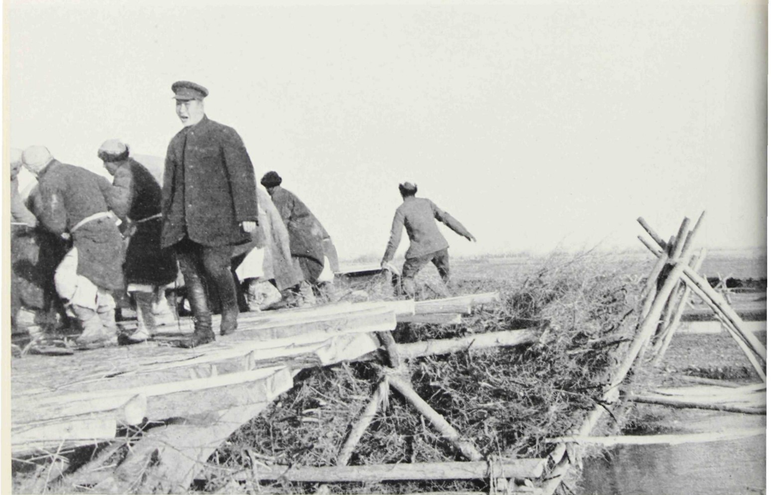
Towing a Truck on to the Aksu River Bridge : Back View of Serat Directing Operations
