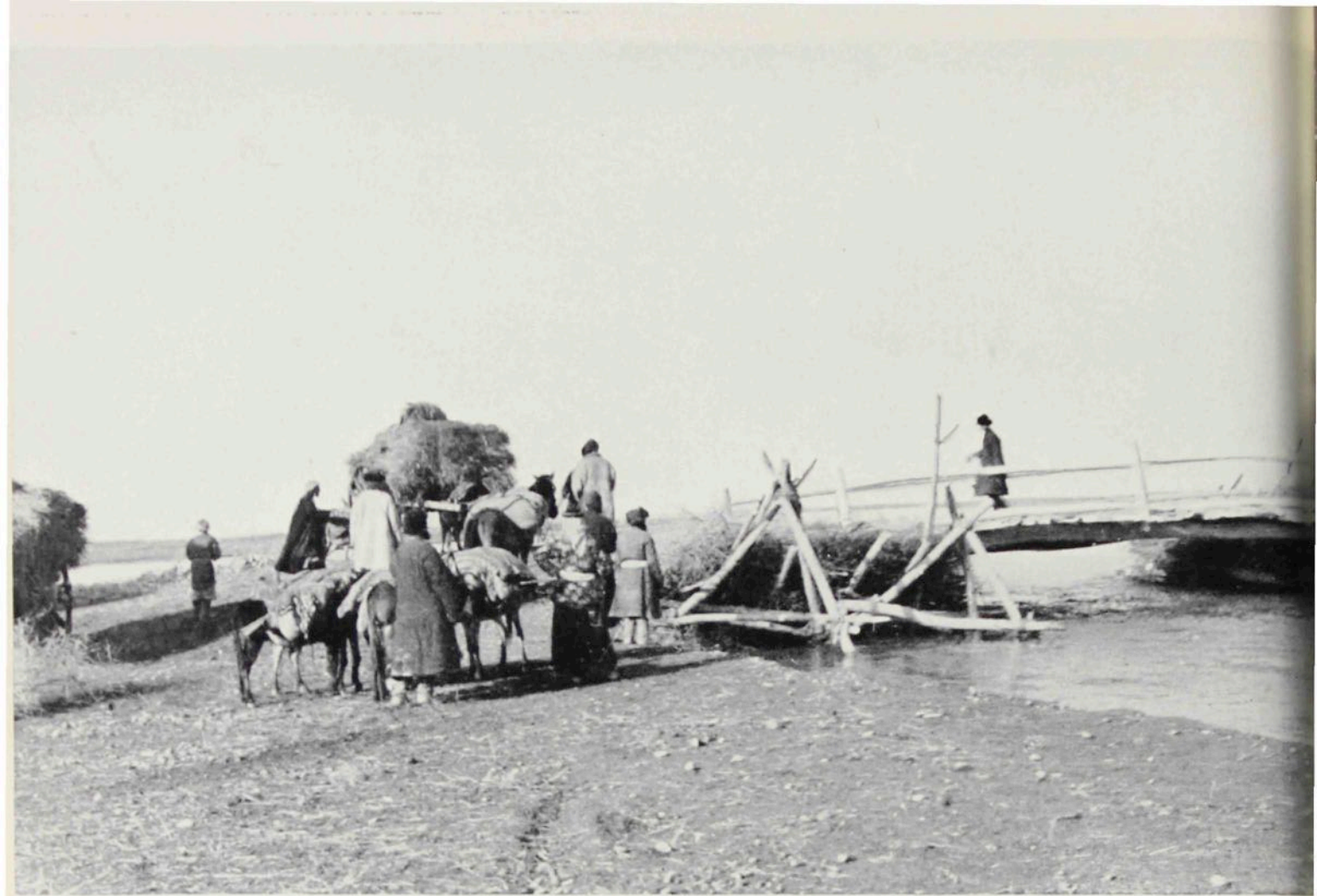
Bridge Over the Aksu River
