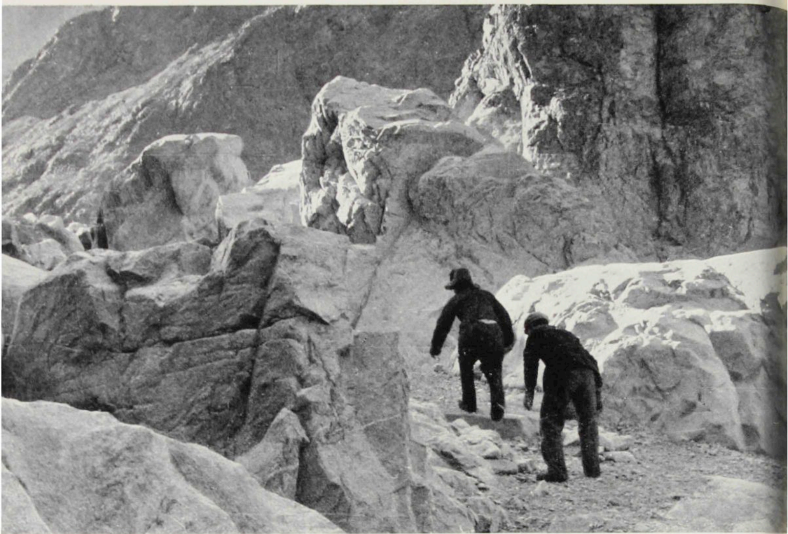
The Rock Passage in the Toksun Gorge : Working on the Road
