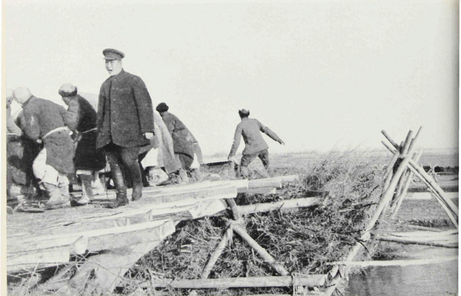
Towing a Truck on to the Aksu River Bridge : Back View of Serat Directing Operations
