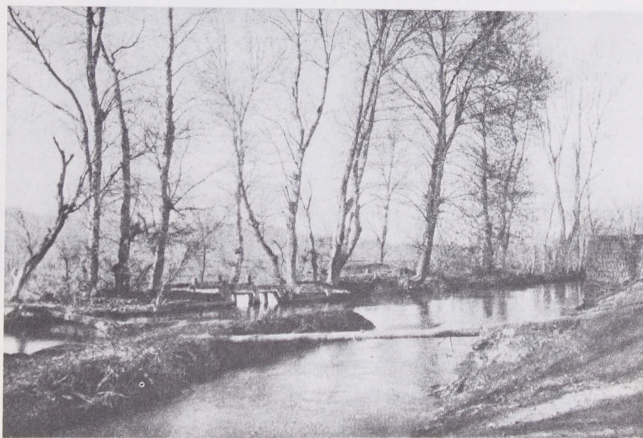
The Urumchi water conduit
